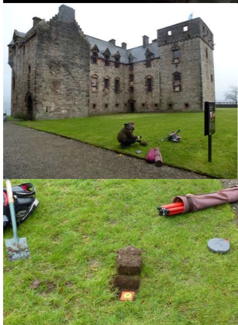
PSMs installation-Providing fixed survey control network with which to align all future survey work.
